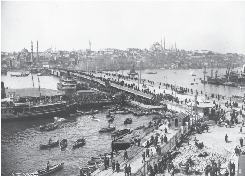
The steel Galata Bridge after it had been built in 1913 © German Archaeological Institute (DAI), Istanbul
